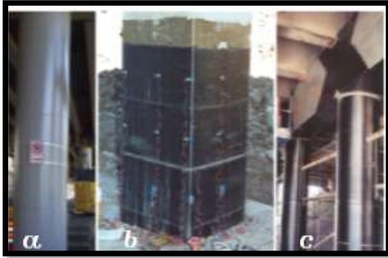
Figure (1): Column jackets: (a) steel, (b) CFRP square, (c) CFRP circular 2. Forward Kinematics Modeling
