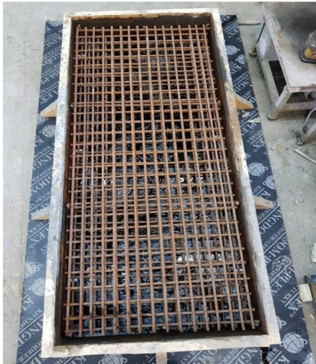
Plate 1 Solid Slab with Top and Bottom Steel Mesh
