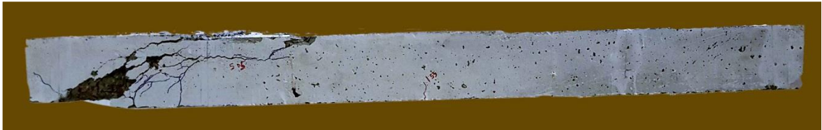
Plate 10 Crack pattern and mode of failure of bubbled slab (G4-S1)
