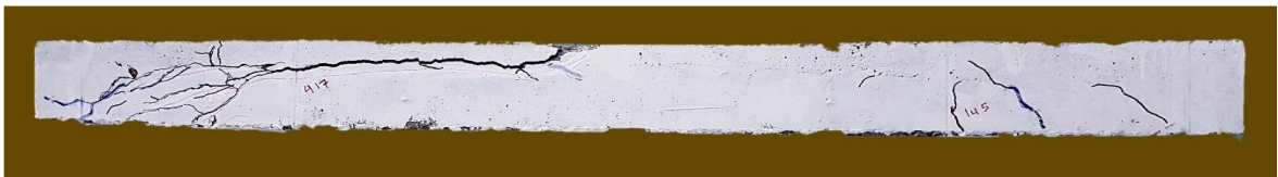
Plate 15 Crack pattern and mode of failure of bubbled slab (G5-S2)
