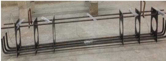
Plate 3: Steel cage of beam ( $B_2$ )
