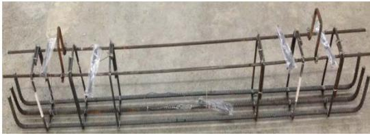
Plate 2: Steel cage of beam ( $B_1$ )
