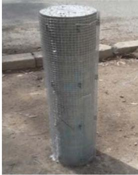
Figure (6): Ferrocement application around the column
