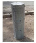
Figure (6): Ferrocement application around the column
