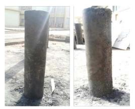
Figure (5): Welded wire mesh wrapping around the column
