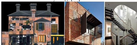
Figure (5): The image shows the stairs and railings reused as a hanging chandelier in the space and highlights the windows installed as a light wall. (Right), the recycled metal doors used on the facade as a privacy and sun-shading device (Center), the reused bricks on the rear facade reassembled in a surreal manner. (Left), source: Peter Bennetts Photographer, 2013.
