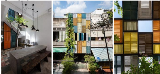
Figure (8): Reused wooden window shutters on the facade of the new house. (Right, left, center) [39]
