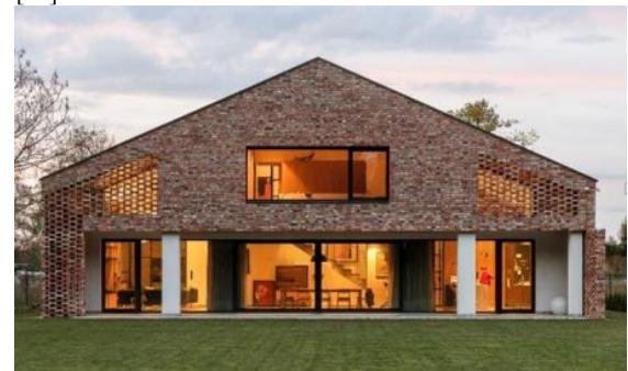
Figure (10): A new house made of old bricks in Poznań, Poland, recycled bricks designed by. Architecci W [33]
