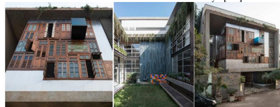
Figure (6): The picture shows the doors and windows from the old houses of the city of Nephi, which were reused in the front facade of the house (right, left), Remnants of metal pipes are grouped together like a bamboo “wall of pipes” merging structural columns and rainwater drainage pipes together (center). Source: [37]
