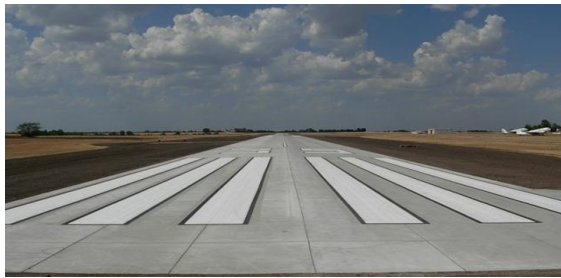
Figure (4): Rigid Pavements
