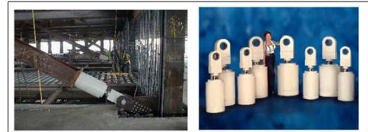
Figure 8: Dampers installation in Torre Mayor, source [12]
