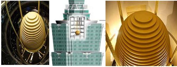
**Figure 11:** Location of Taipei 101's largest tuned mass damper. source [13]
