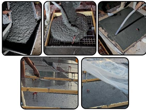
Figure (6): Concrete casting
